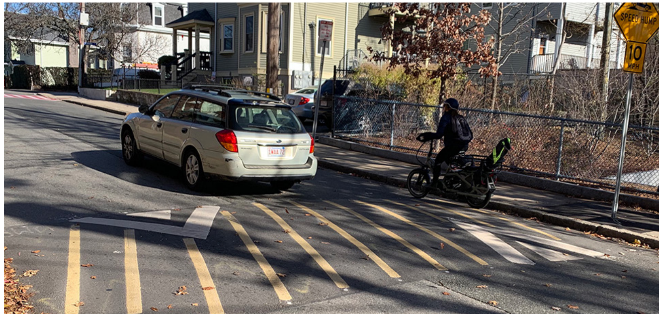
One of a series of speed humps on Central Avenue in Somerville, MA.
