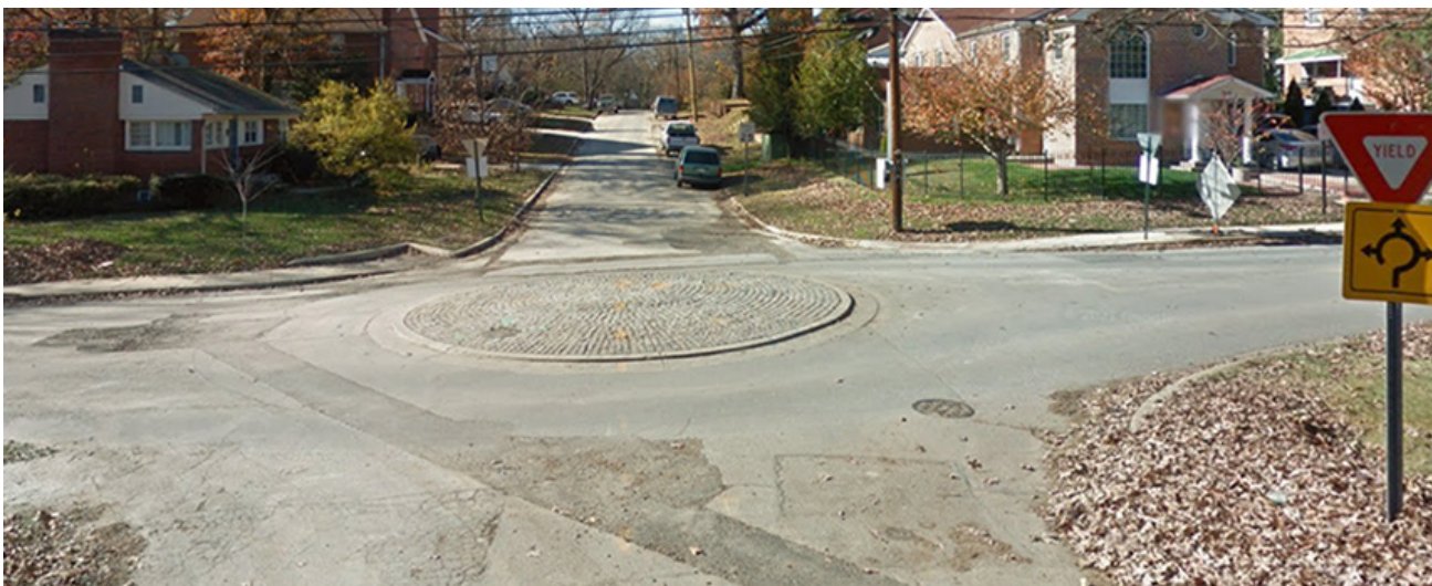
Traffic calming roundabout
