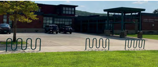
MAUMS bike rack is a Wave Rack which only supports the bike frame in one location and is not recommended.
