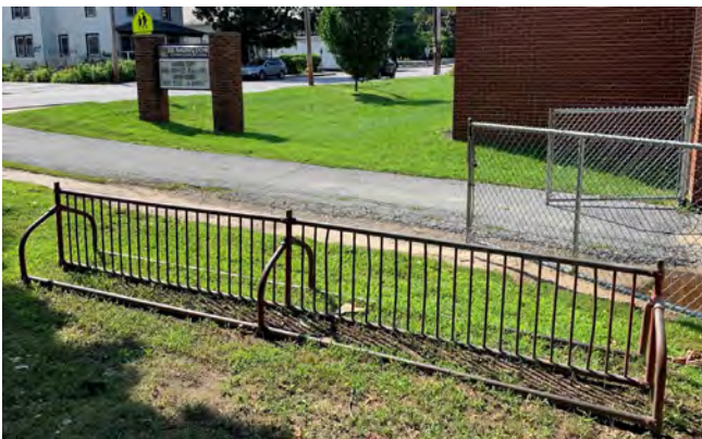
Bennington Elementary's bike rack does not allow locking of the frame and can cause front wheel damage.
