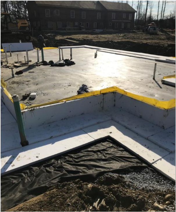
FPSF with insulation "wing" installed to extend frost protection to the soils under the slab edge.
