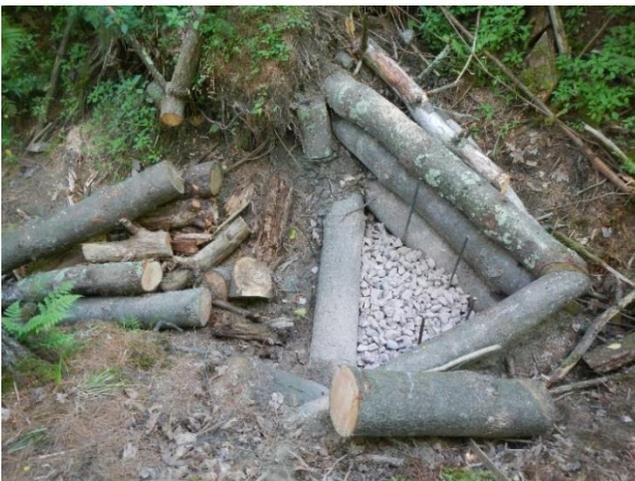
**Figure 3:** “V-type” log check dam designed and installed by FEA on a gully in Colchester, VT. Flow is from right to left.
