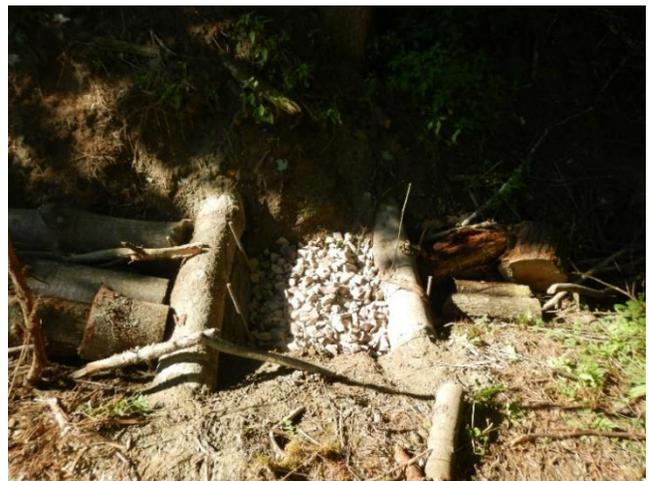
**Figure 4:** “Straight” log check dam designed and installed by FEA on a gully in Colchester, VT. Flow is from left to right.
