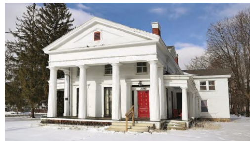
The future site of Bennington Family Housing. Courtesy of Shires Housing
