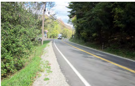
There is no good place to walk for a short, critical stretch along VT 7A.
